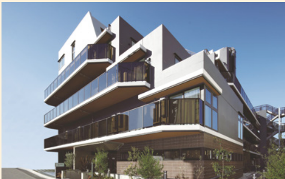
Exterior of "Granda Yotsuya"
