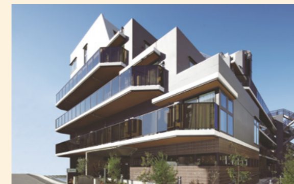
Exterior of "Granda Yotsuya"
