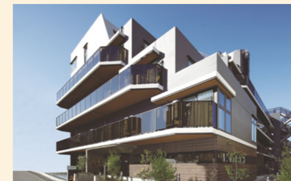
Exterior of "Granda Yotsuya"
